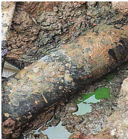
Force main break at the Hallmark Lift Station
