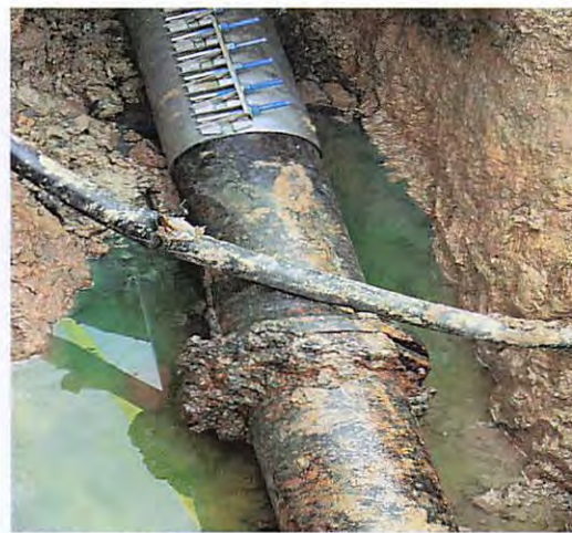
Force main break at the Hallmark Lift Station
