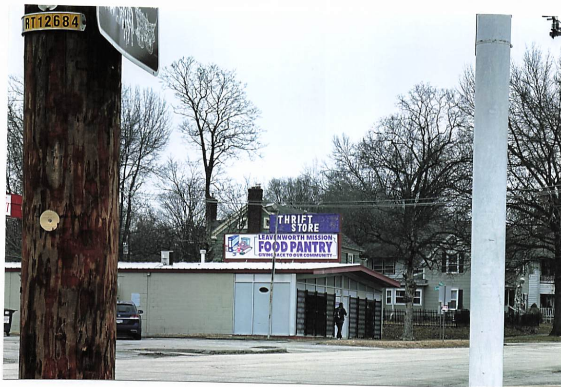
South side of building
