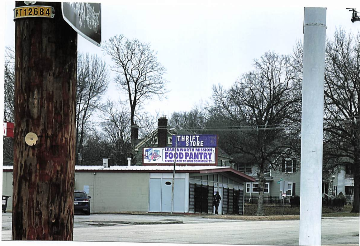
South side of building
