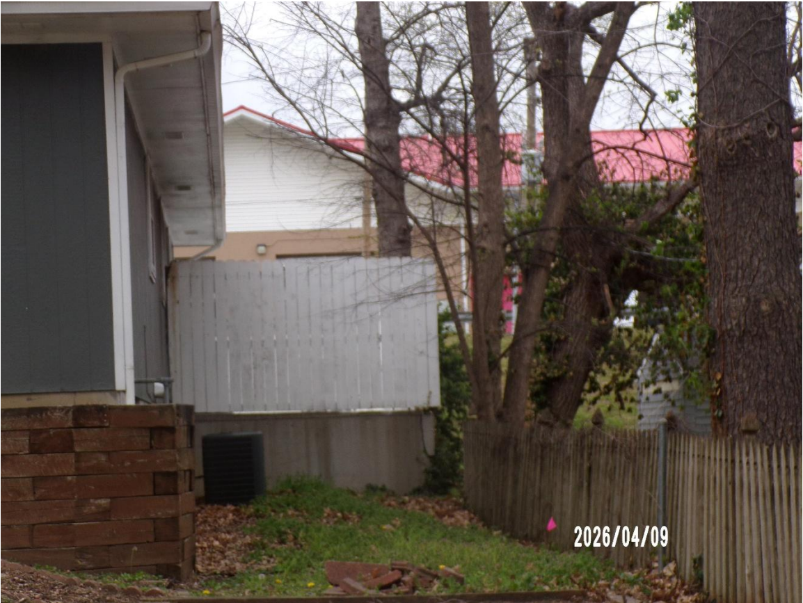
Facing north from the front yard (current 6-foot fence)
