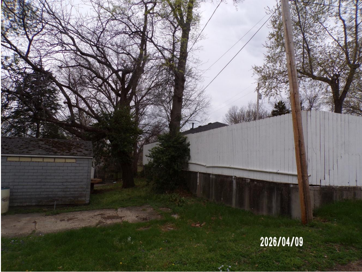
Current 6-foot solid fence on the east property line
